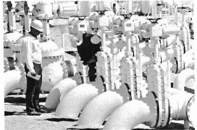
Capline was built to supply crude oil to refineries in the Midwest. Although pipes, valves and meters are visible (right), most of the system lies buried out of sight. Inside the station at Patoka—the northern end of the line—a wall-to-wall monitoring panel is kept under surveillance around the clock.
