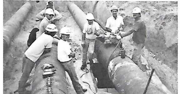
"Man, I hope they don't forget we're down here and backfill."
