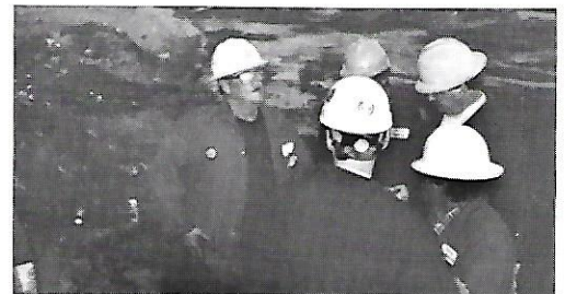
Jim Avery and crew prepare to make repair.
