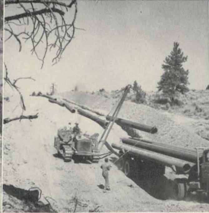
MILE AFTER mile the Butte line stretches giving the reader a good idea of the land through which the pipe goes. R. E. Shaw, who worked on the line as a right-of-way man, uses binoculars to check for incoming supplies. Above, men put down sections of pipe along the right-of-way in one of the early stages of laying the line in the hot, dusty country.
