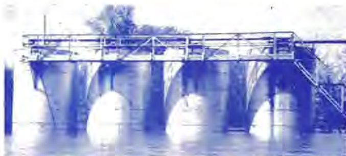
Tanks mounted on 8-foot piling in Deep Fork River Bottom.
