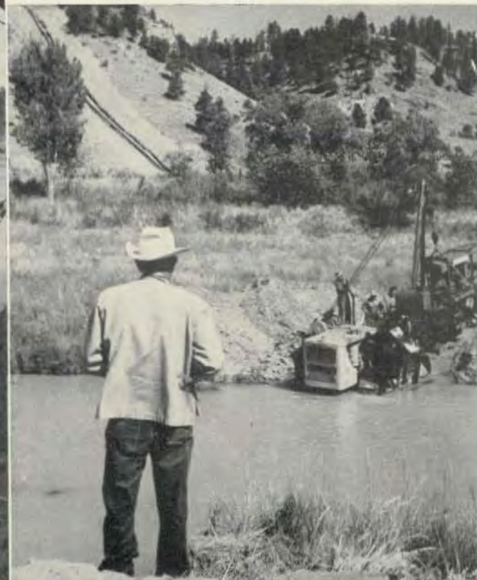
MISSOURI RIVER crossing was accomplished (left) when the Fort Peck Dam spillways were shut down to allow the men to work in shallow water. Cooperation like this was sincerely appreciated by the construction crews. The crossing was near Poplar, Montana. Below, a worker watches as a crew starts to move equipment over the Belle Fourche River. Forging the river meant saving 34 miles in moving equipment to the line which can be seen in the left background on the hillside.
