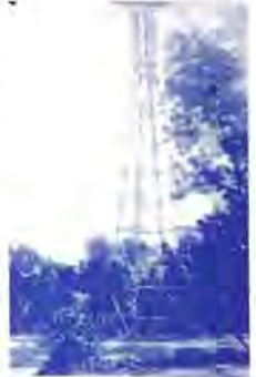
Last picture taken of T. & T. Red River crossing tower which location at height of flood was 400 feet out in channel. The tower was washed away as were 27 of the poles on the south side of the river.
