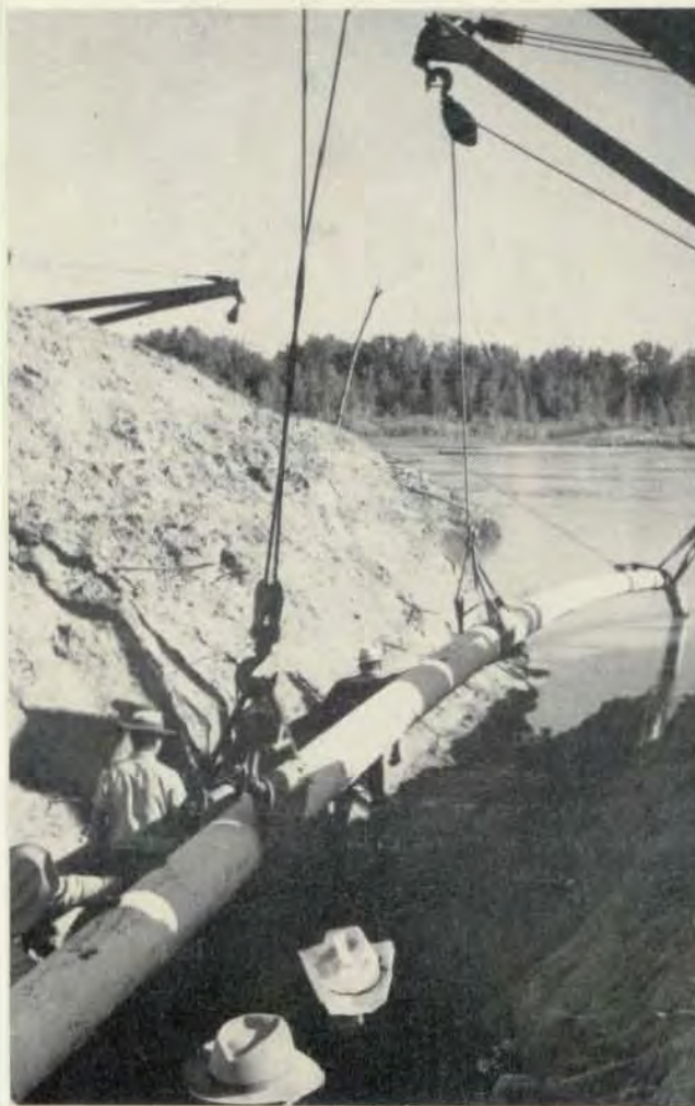
MISSOURI RIVER crossing was accomplished (left) when the Fort Peck Dam spillways were shut down to allow the men to work in shallow water. Cooperation like this was sincerely appreciated by the construction crews. The crossing was near Poplar, Montana. Below, a worker watches as a crew starts to move equipment over the Belle Fourche River. Forging the river meant saving 34 miles in moving equipment to the line which can be seen in the left background on the hillside.
